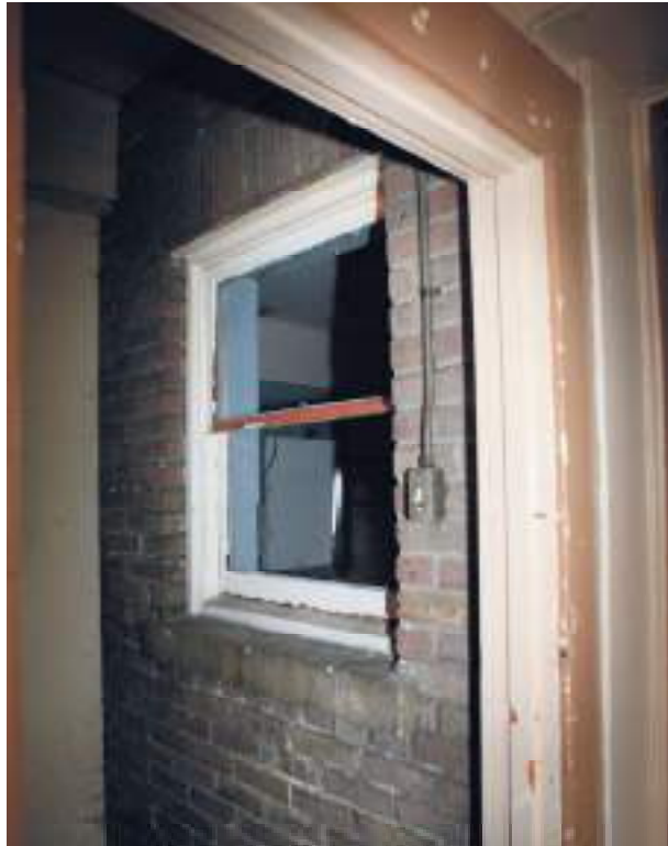
CP13. Detail of original west exterior and window; now housed within small 1-story addition, NW corner of building.
